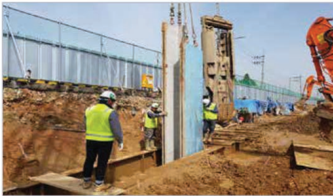
3. BOX-TYPE구간 PC-WALL 근입
